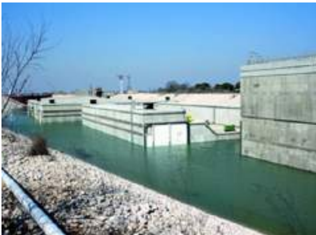
Caissons made of reinforced concrete form the foundation of the flood protection system
