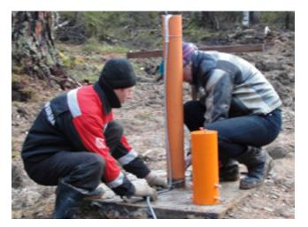
Installation of level tubes at hard-to-reach locations
